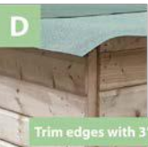
Neaten & cut excess felt
